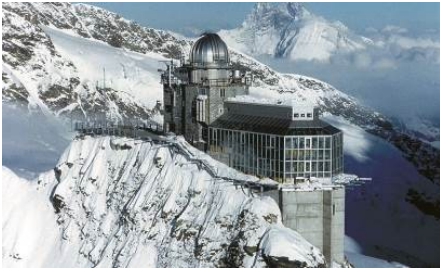
Fig. 1: insulbar insulating profiles successfully protect the mountain-top "Sphinx" restaurant on the Jungfrauoch from temperatures as low as -30°C and wind speeds of up to 250 km/h.
