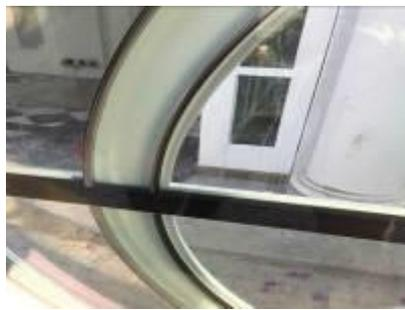
Pictures 3 and 4: Installation of the new safety glass doors and windows: Window constructor LIP-GmbH used double insulated glass from Nowak Glas with Thermix Warm Edge spacers and muntin bars. Picture courtesy of: FAR Frohn & Rojas
