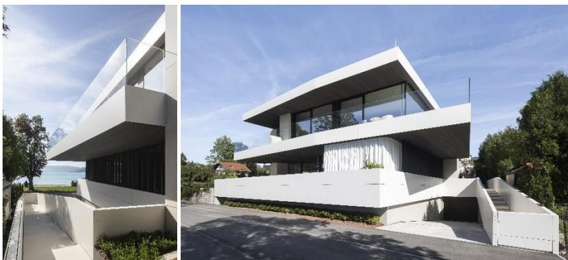
Figs. 4 and 5: The balustrades were also made with Dekton Zenith in a thickness of 1.2 cm. A nice detail: sheet metal cladding on the parapets was not necessary.
