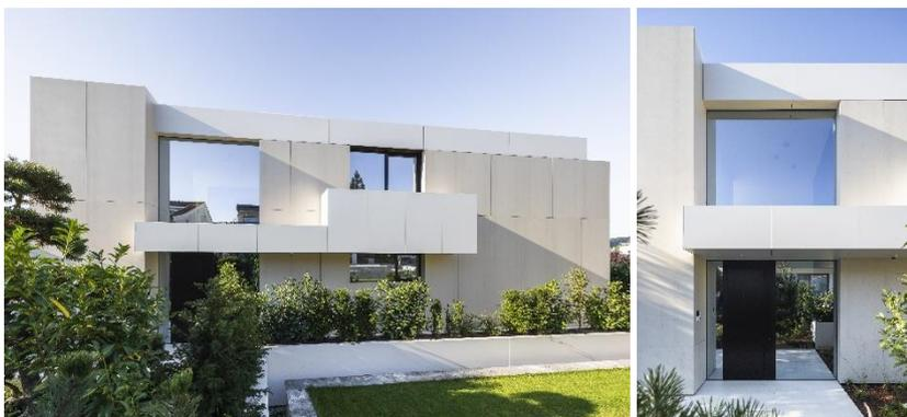
Figs. 2 and 3: The ventilated curtain wall consists of 1.2 cm thick Dekton by Cosentino in the shades Danae on the vertical and Zenith on horizontal elements.
