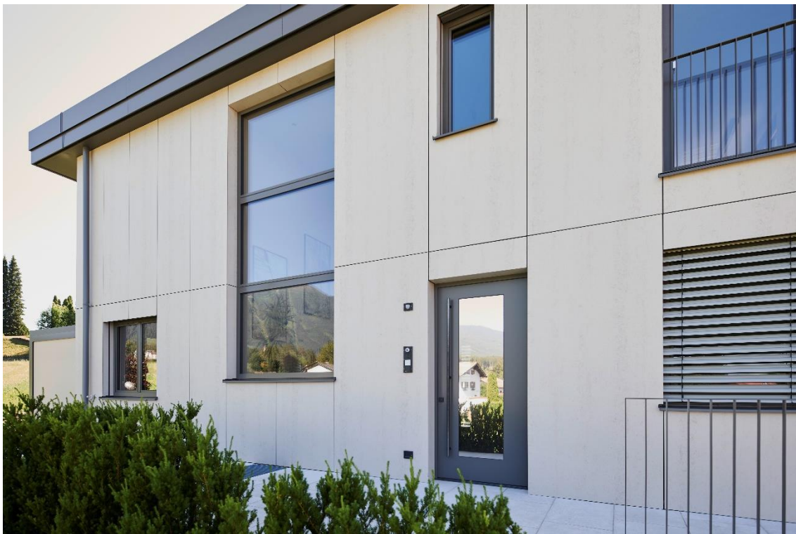
Fig. 3: Story-high facade elements allow the design of an almost monolithic building envelope with a perfectly balanced joint pattern.
