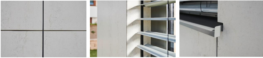
Figs. 4, 5, 6: Maximum precision in cutting the panels is evident from the narrow joints and the exact cut-outs, for example for the roller shutter rails or window sills.
